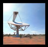
SKA1-SURVEY (ASKAP — Western Australia 36 12-m with Phased Array detectors 700 MHz to 1800 MHz)
