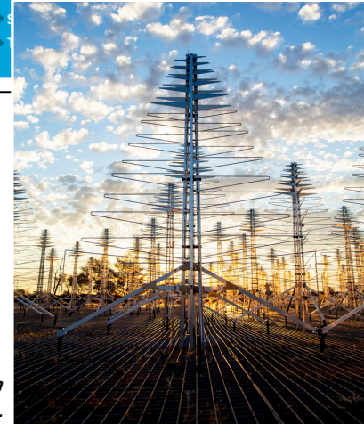
SKA-LOW Prototype station Antenna design SKALA 4.1AL
