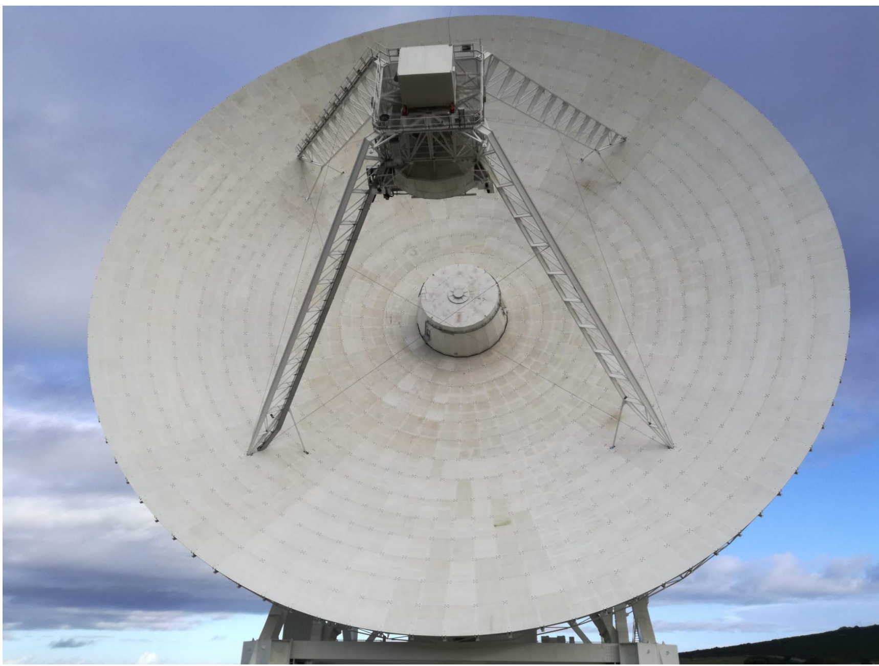
Fig. 1 - Sardinia Radio Telescope Main Reflector (M1). The active surface (AS) allow to modify the shape of the mirror to maintain the profile always close to the ideal one.
