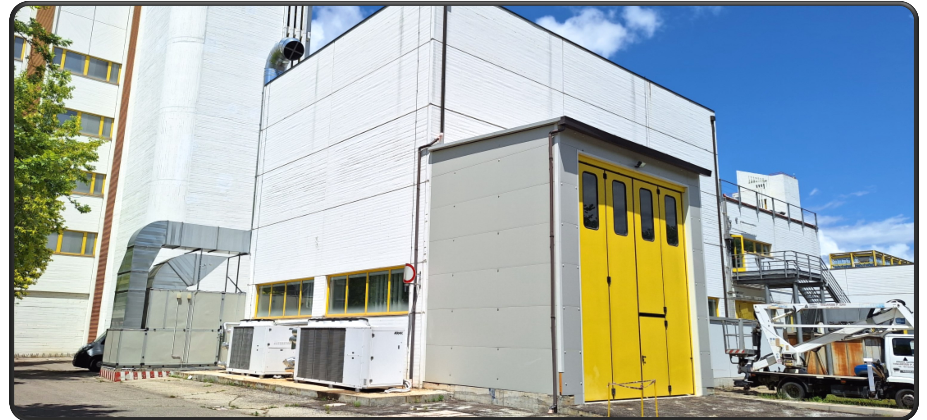
The Bologna Integration Hall, a building of 17.4 x 11.9 x 11.9h m
