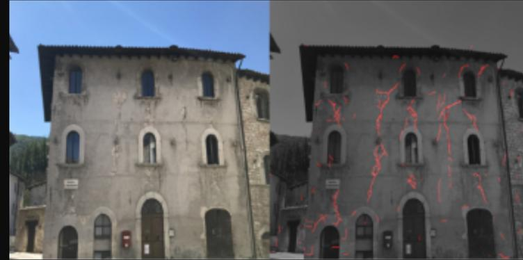
Example of earthquake crack detection, from Pantoja-Rosero et al., 2022
