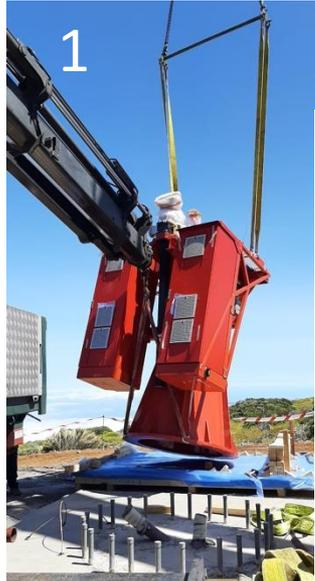
1. Install the telescope base, that includes the AZ fork & AZ motors, the electric cabinets and the EL actuator
