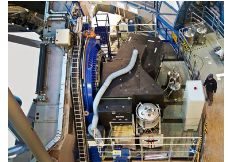
SPHERE installed on VLT Credit: ESO / J. Girard
